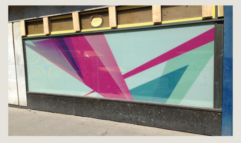
The fitting process had two stages. Before the installation could take place, the existing film had to be removed from the glass. The work was undertaken by one of The Window Film Company's experienced and fully qualified fitting teams, who removed the film carefully but efficiently, ensuring that the surface was clear and clean ahead of the fresh installation.
