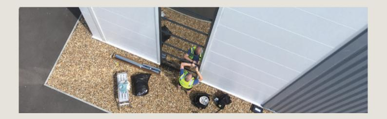
The nature of the building meant that an internal application of the film wasn't possible - large storage racks prevented the necessary access to the glass. In addition, many of the affected panes, of which there were 48, were at a height that necessitated powered access equipment to reach them. Using this sort of equipment inside the premises would have created too much disruption to daily operations and so an external installation was agreed.
