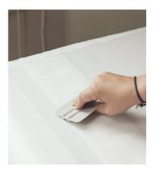
Card over the design using the Squeegee supplied to increase the bond between the application tape and Frostbrite® film
