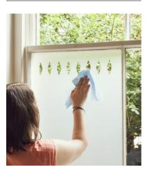
Finally wipe off any remaining water from the film and the frame being especially careful around the edges of any cut outs not to lift the film
