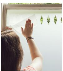
Once dried for 24 hours, spray the application tape lightly and leave to soak for 5 minutes. Slowly peel off the application tape making sure you keep it close to the window, this will then reveal the design
