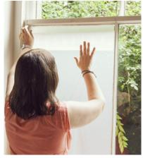
Take the film to the window making sure you keep it taut, allow the film to flow onto the glass and slide into position
